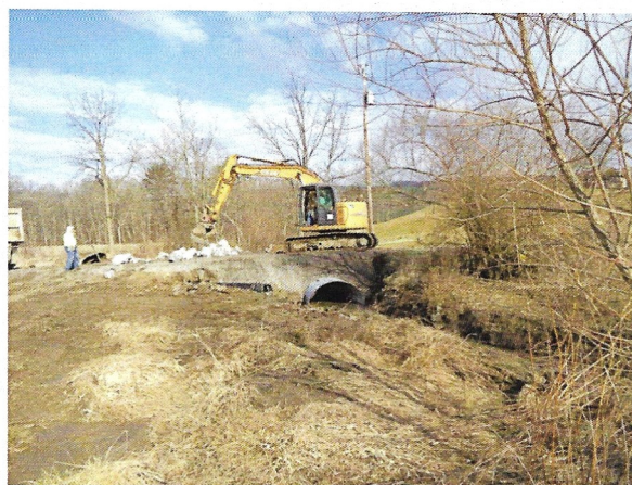
Putting in the culvert on Blair Road.
